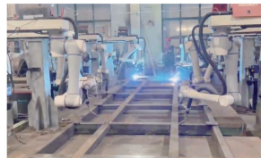
Steel Frame Welding
